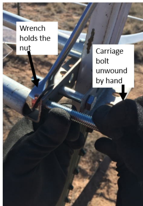
Figure 2: current way to remove rainout panels via carriage bolts
